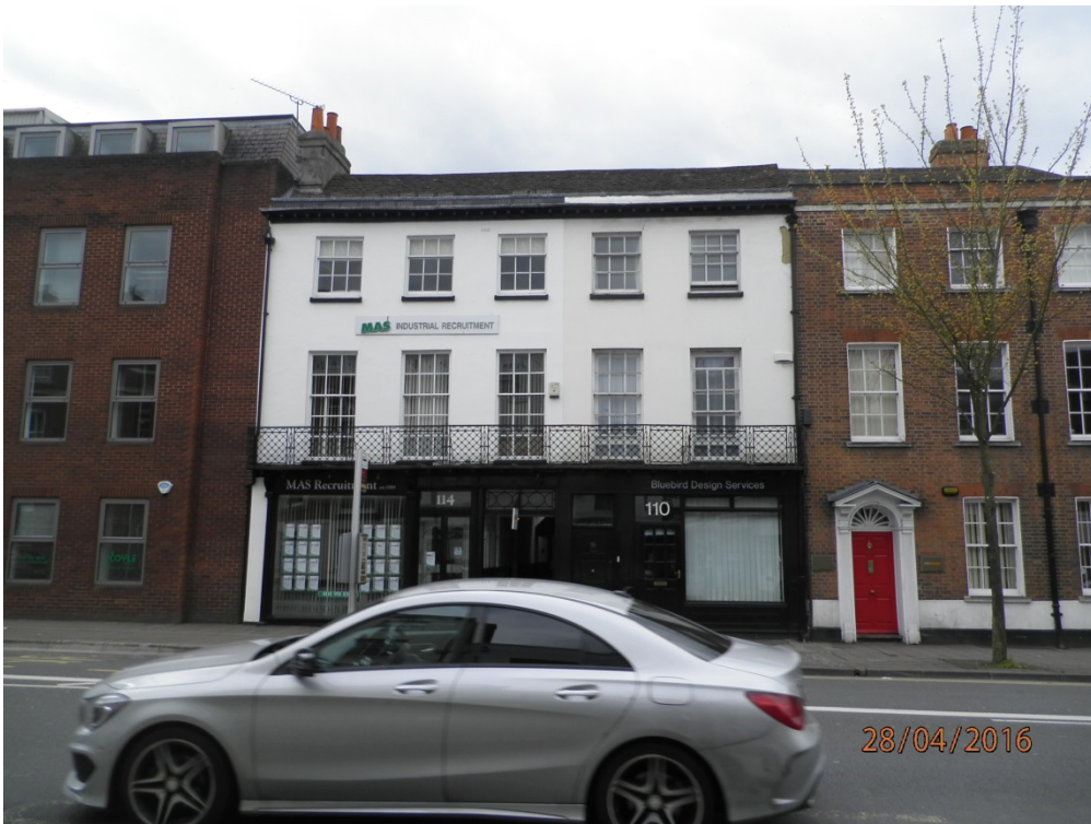
Listed Buildings at 110 and 114 London Street, with passageway entrance to the After Dark Club in the centre of the building
